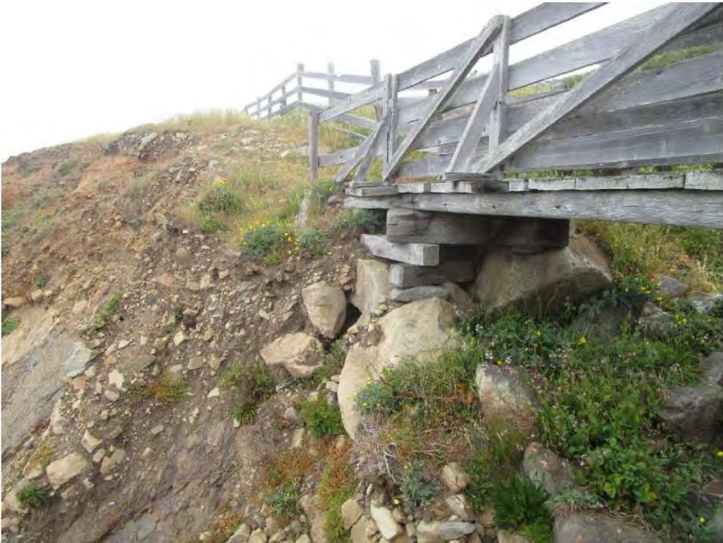
BRIDGE 2 NORTH ABUTMENT, LOOKING NORTH
