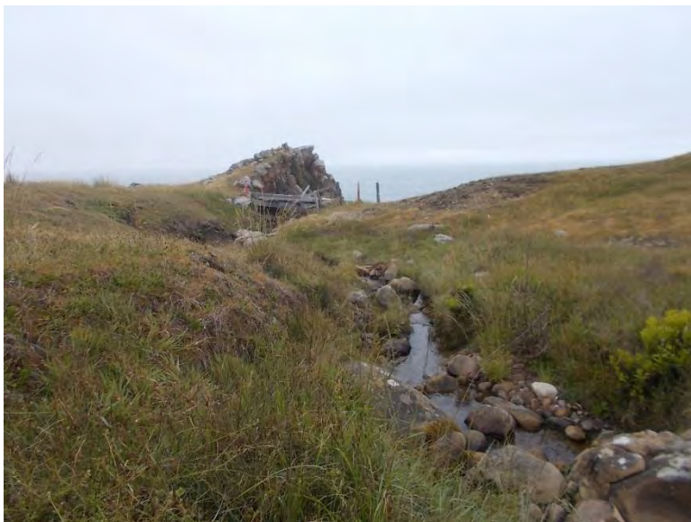
PHOTO 2: DRAINAGE D-5 WITH FRINGE WETLANDS LOOKING WEST TOWARDS OCEAN. COLLASPED OLD WOODEN BRIDGE IN BACKGROUND.
