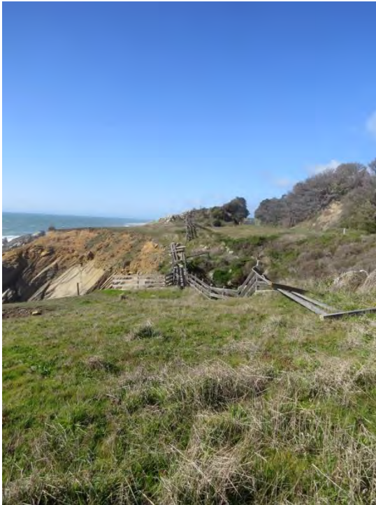
Photo 1 - Historic Wooden Bridge
