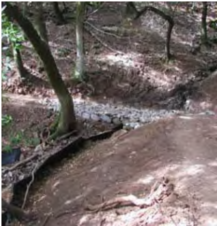
Image 44. Armored crossing. PHOTO: REGIONAL PARKS
