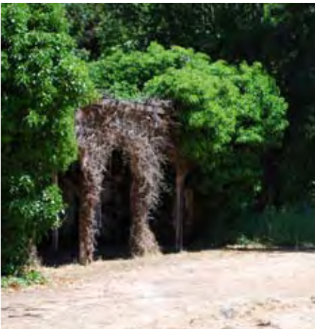
Image 58. Garage/stable. PHOTO: RRM
