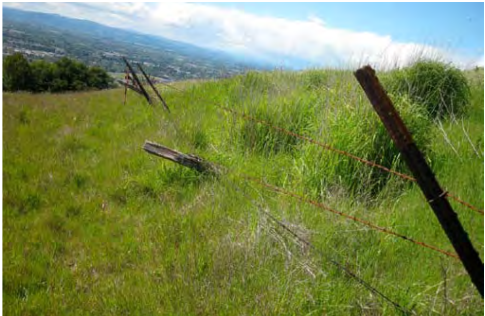
Image 18. Boundary fence in need of replacement. PHOTO: LISA BUSH
