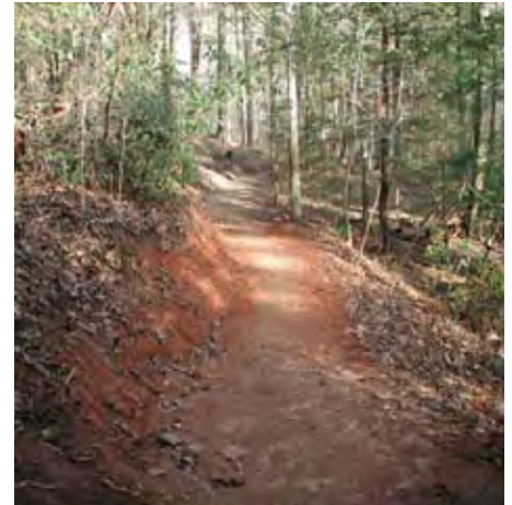
Image 40. Full bench trail construction. PHOTO: I.M.B.A.
