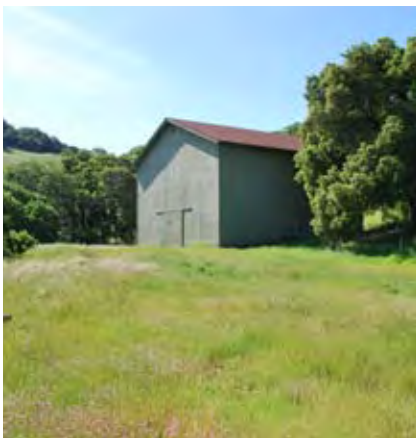
Image 70. Existing barn. PHOTO: RRM
