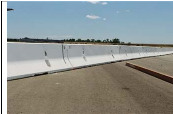
Type 60 Concrete Barrier (K Rail)
