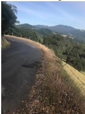
Los Alamos Road (12 feet wide for last mile)
