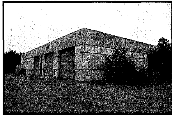
Service Center – Front Exterior
