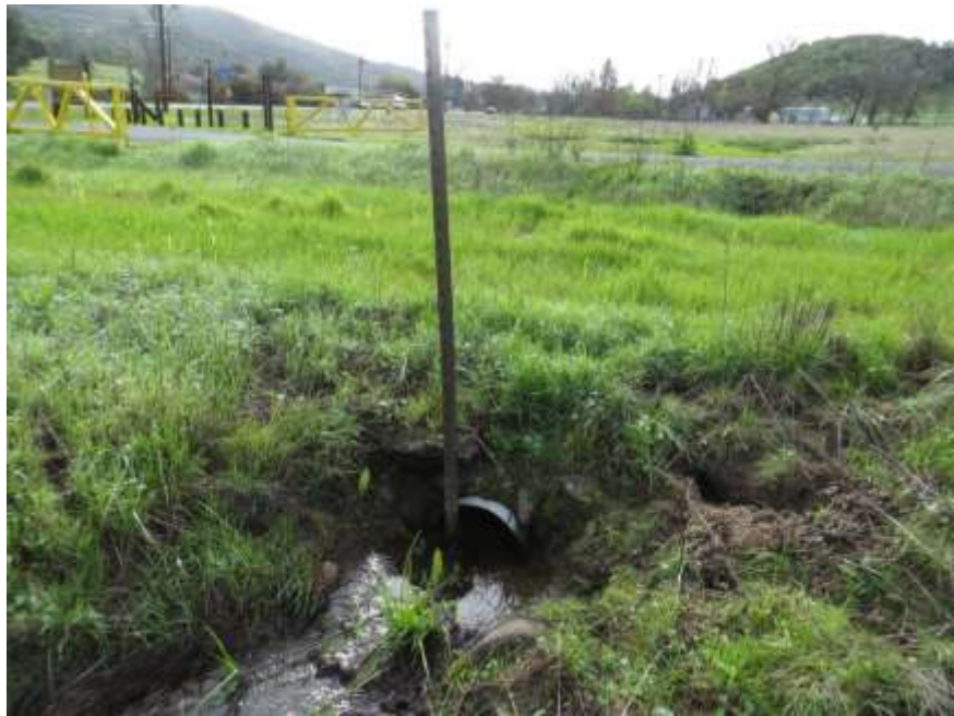
Culvert under old ranch road on Curreri.
