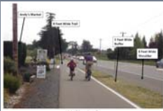
Looking South West County Trail paralleling Highway 125 near Sebastopol
