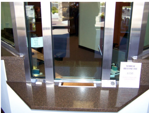
Example of Security Window in Lobby Can be difficult to communicate through
