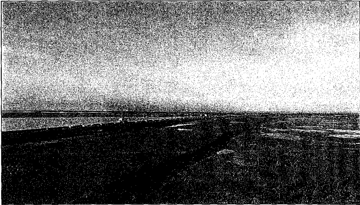
Setback levee built to protect SR 37 for the Cullinan Ranch tidal marsh restoration project, part of the USFWS San Pablo Bay National Wildlife Refuge. (Photo: Ducks Unlimited)
