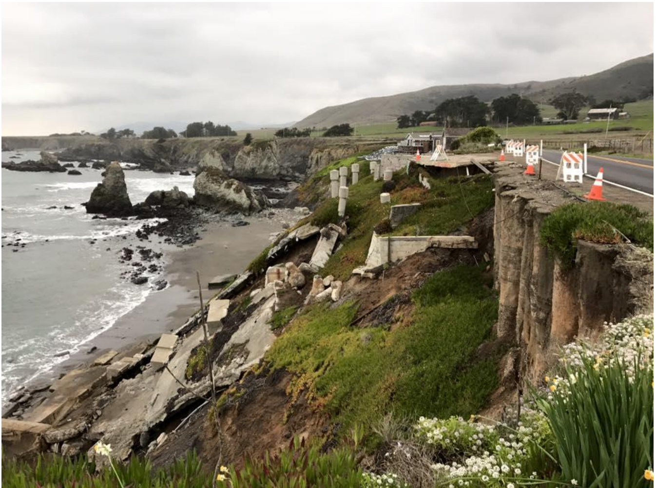
Caltrans Work Area – Gleason Beach
