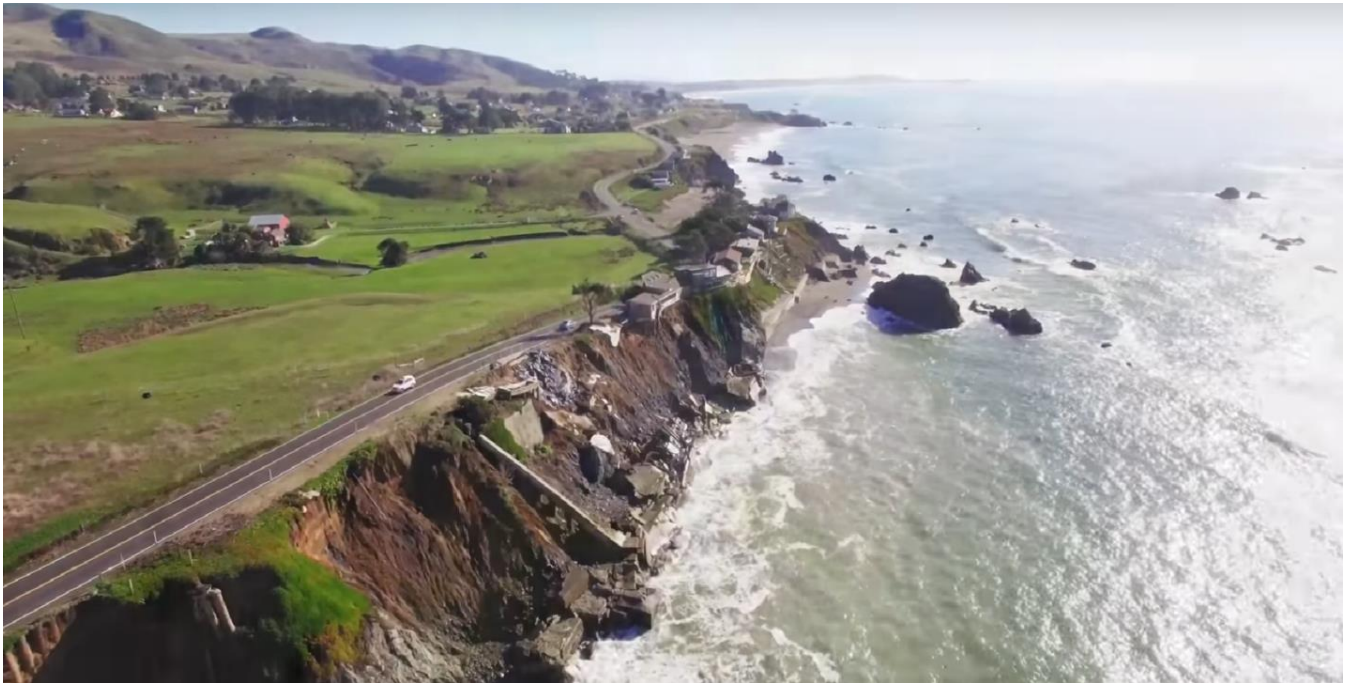
Debris on Beach, Northern Aspect – Gleason Beach
