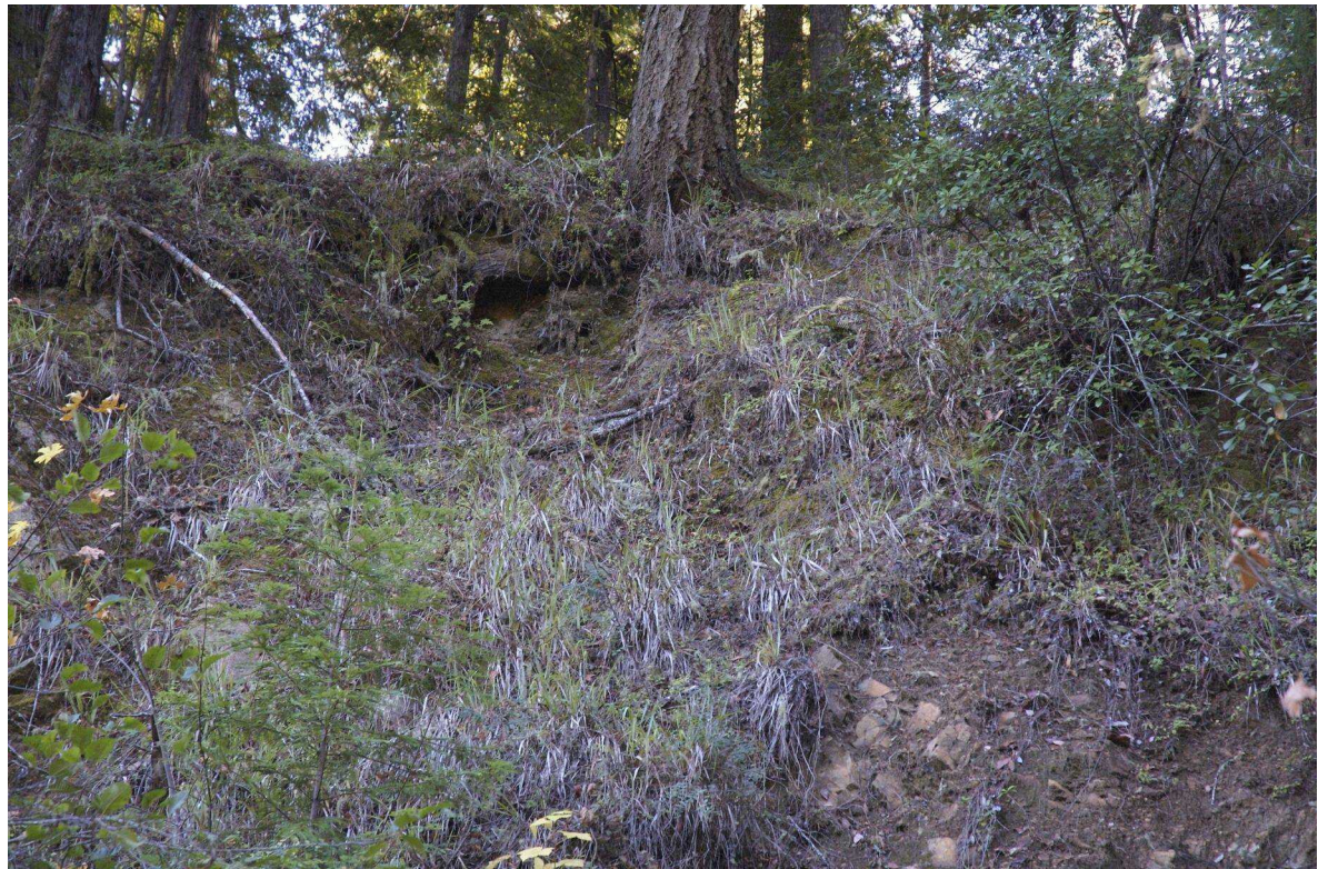
These photos show the top of the landslide area where trees have been undermined and “left hanging,” so to speak.
