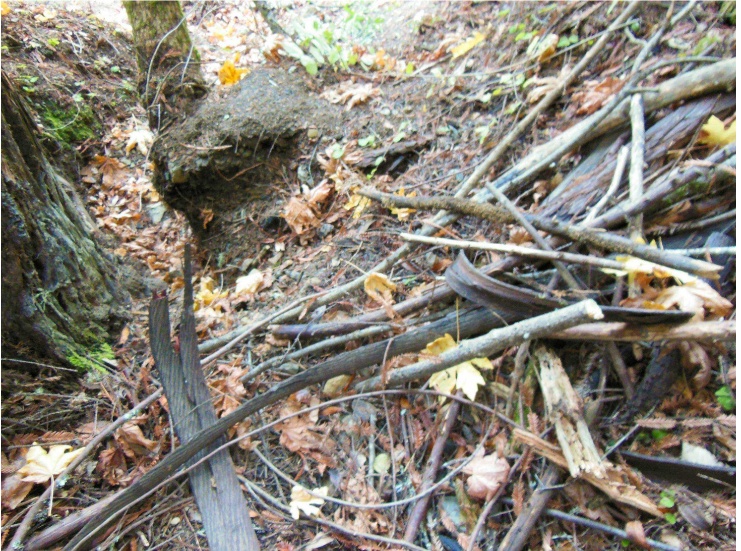
Branches have collected at the road end of the ravine, carried downhill by water.
