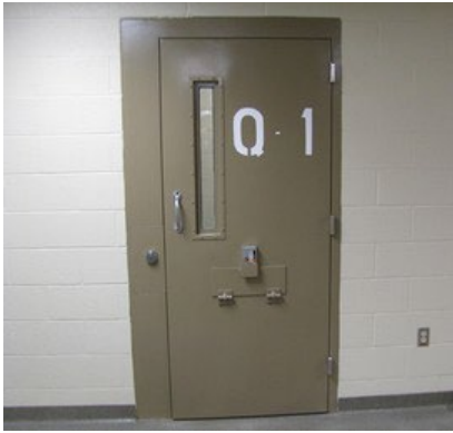
Sample of Door- 26.5 lbs. Pull Force A Module
