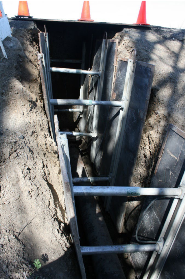
Example Photo 5: Shoring Site Safety Analysis/SOP Development/Safety Training
