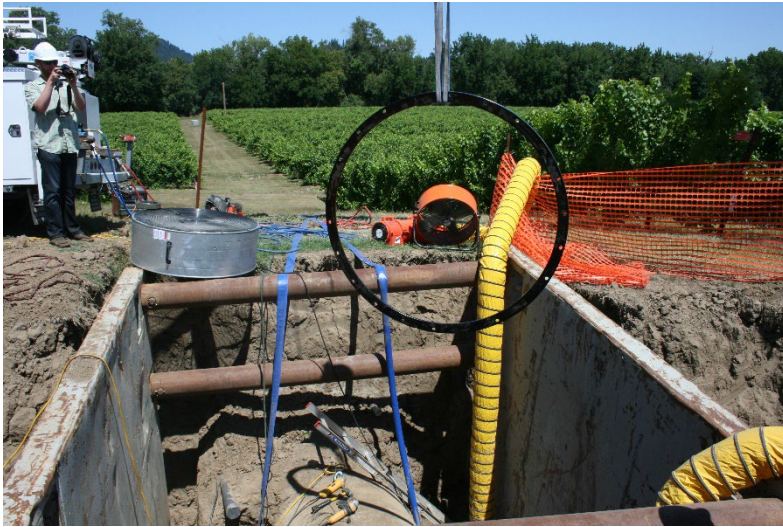
Example Photo 1: General Construction Site Safety Analysis
