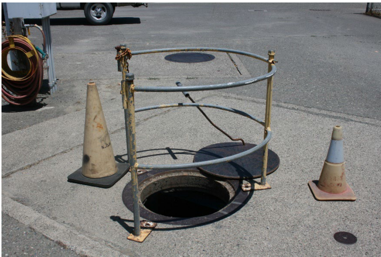
Example Photo 2: Inspections/Safety Trainings Involving Removal of Street/Manhole Covers
