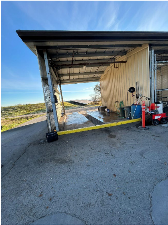
Vehicle/Equipment Wash Bay
