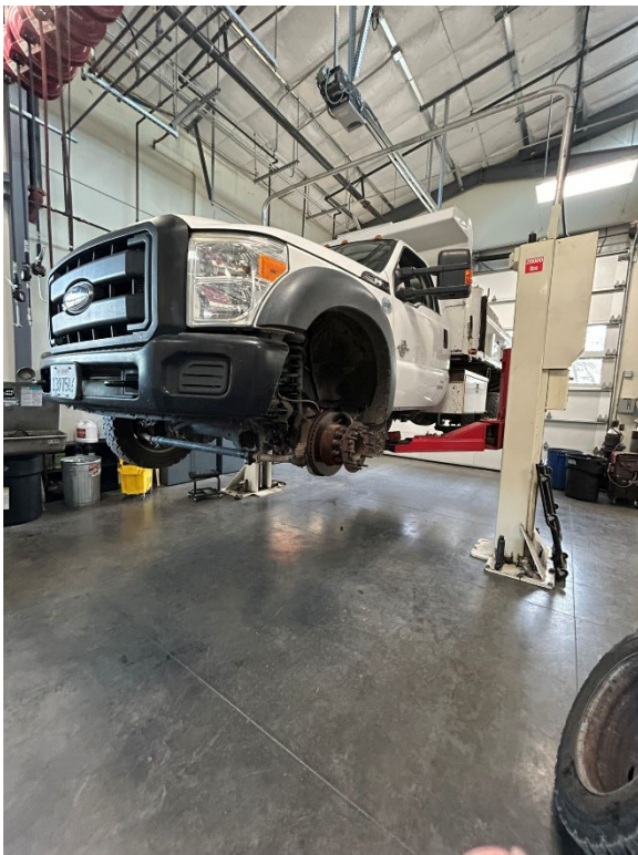
Truck on Lift for Brake Repair
