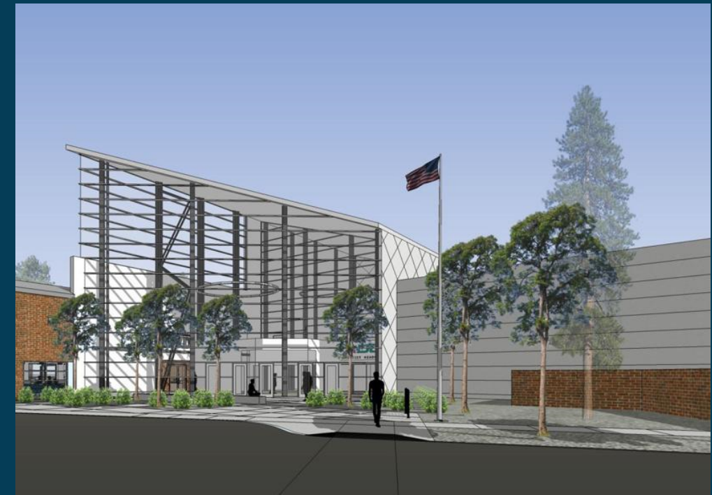
ARIZONA DEPARTMENT OF TRANSPORTATION FLAGSTAFF FACILITIES
