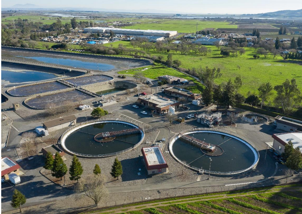
Sonoma Valley Wastewater Treatment Plant
