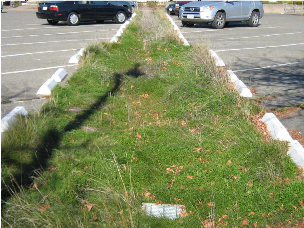
A vegetated swale in the P.R.M.D. south parking lot filters urban runoff
