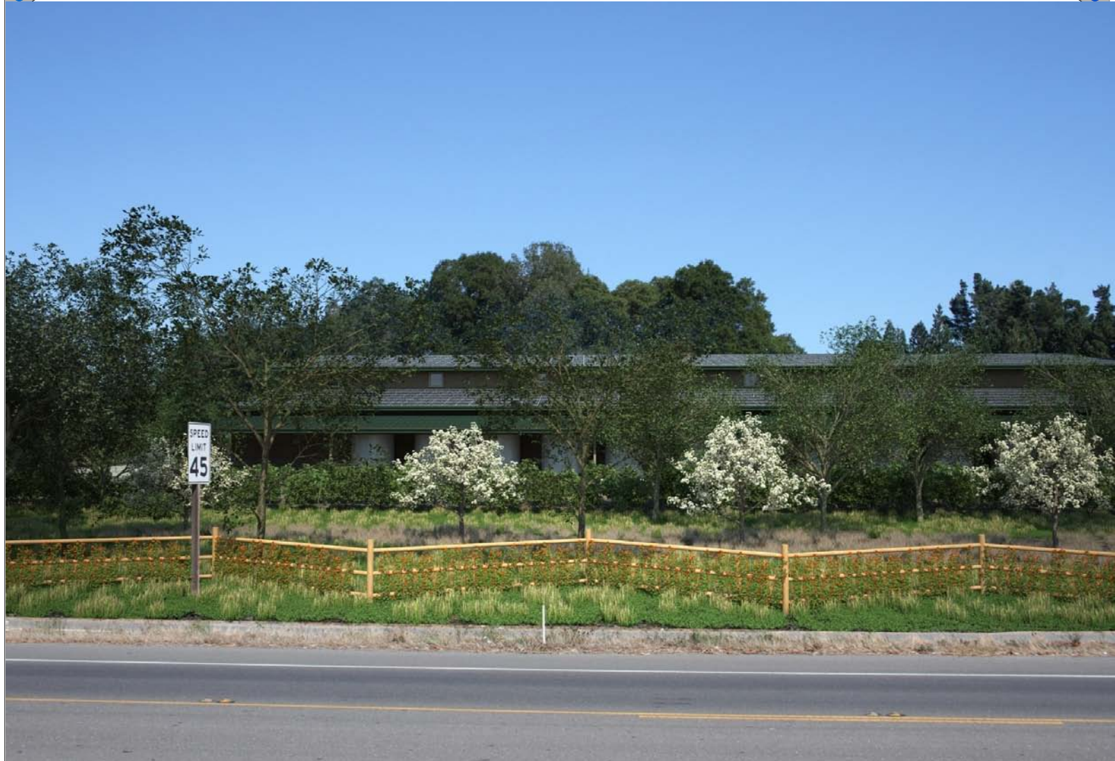
View (4)- Frontage Hwy 116- mid section of project site
